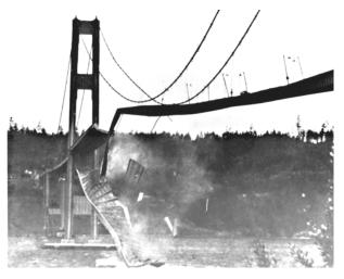
At 10:30 am the oscillations had finally caused the center span floor panel to fall from the bridge. The rest of the breakup occurred over the next 40 minutes.
