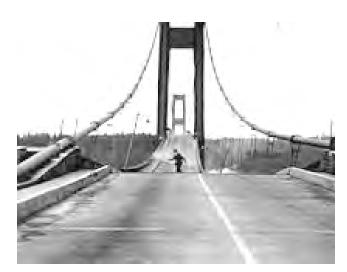
The bridge had a secondary standing wave in the first mode with its one node on the centerline of the bridge. The man in the photo wisely walked along the node. Although the bridge was heaving wildly, the amplitude at the node was zero, making it easy to navigate.
