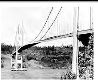
Vortices around its deck caused by winds of 35 - 40 mph caused the bridge to begin rising and falling up to 5 feet, forcing the bridge to be closed at about 10 am. The amplitude of motion eventually reached 28 feet.
