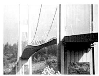
The Tacoma Narrows Bridge on November 7, 1940. Workers on the construction of the bridge had referred to it as "Galloping Gertie" because of the unusual oscillations that were often present. Note nodes at the towers and in the center of the deck. This is the second mode.
